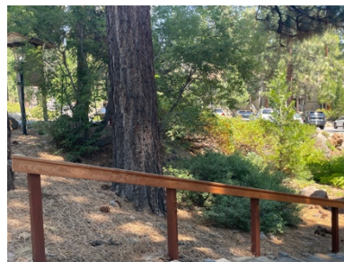
Sturdy new railing
